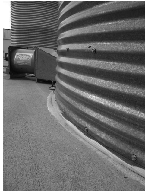
Figure 12. Base of bin sealed with elastomeric sealant.
