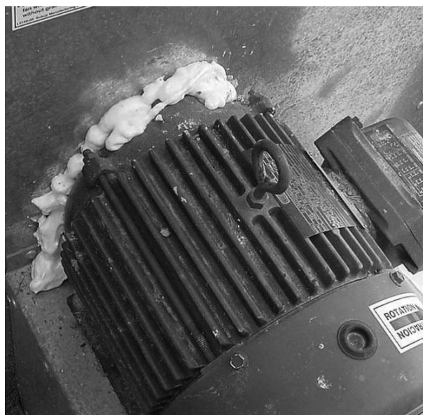
Figure 11. Aeration fan motor housing to fan enclosure sealed with expandable foam.
