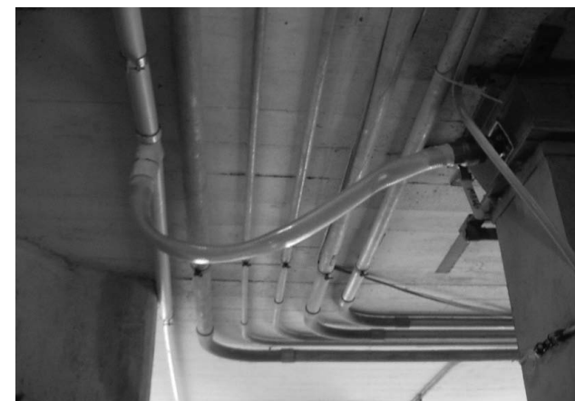
Figure 4. CLF injection point with ball valve into discharge spout of concrete elevator bin.
