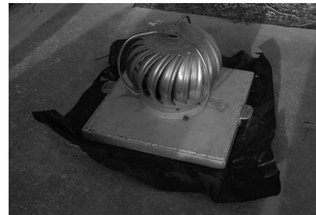
Figure 15. Temporary sealing of ventilation hatch using polyethylene film.
