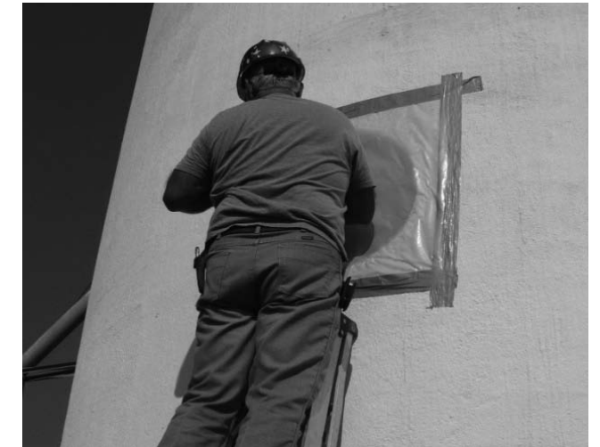
Figure 16. Temporary sealing of hatch on concrete silo prior to fumigation.
