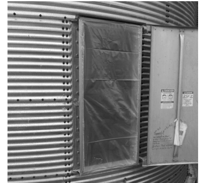
Figure 17. Access door sealed with polyethylene film and duct tape.
