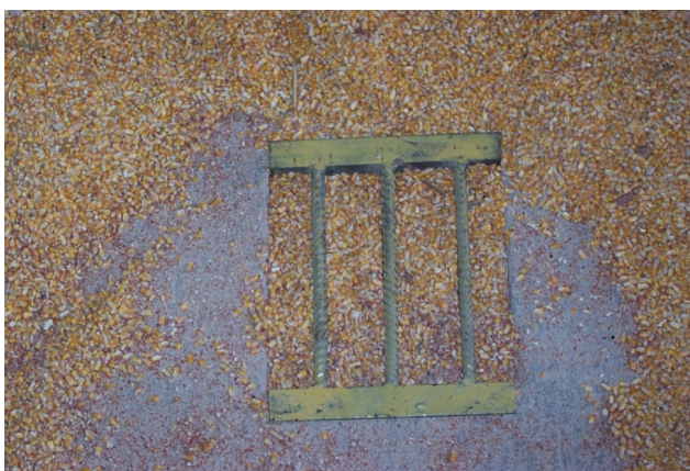
Figure 4. Improperly secured grate.
