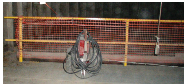
Figure 11. Sweep auger worker protection fencing.
