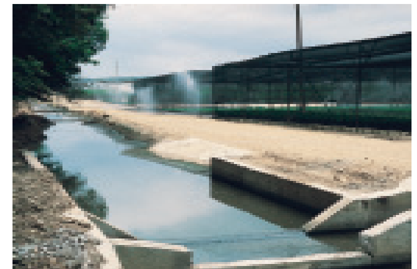
In a capture and recycle system, irrigation runoff from nursery beds and houses in production areas is collected by a system of channels or ditches leading to retention basins.
