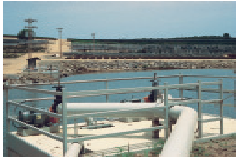
Once irrigation runoff is captured in retention basins, it can be recycled directly back onto nursery crops, diluted with fresh water, treated to remove plant pathogens, and/or stored for future use.
