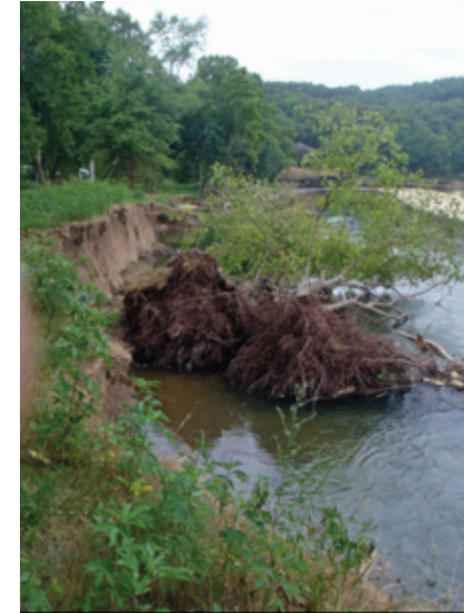
Figure 4. A tree toppling into a river is a sign of a mass bank failure.
