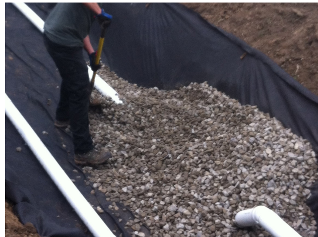
Figure 5. Installation of an underdrain.
