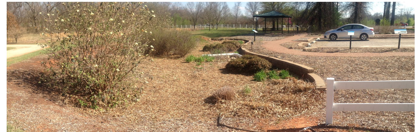
Figure 6. Bioretention cell at the OSU botanic garden.
