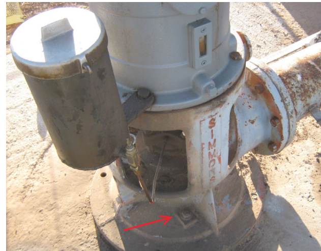
Figure 2. Pump base showing access hole location.
