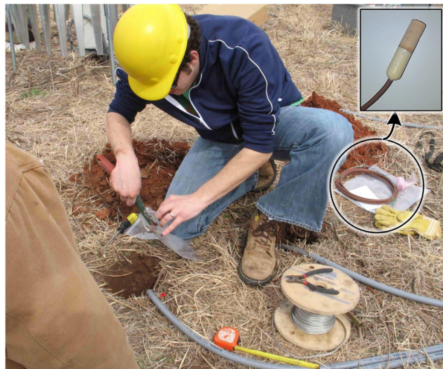
Figure 1. Installation of a soil moisture sensor at a Mesonet site.
