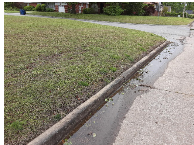
Figure 5. Seepage faces exist at many areas, where the water table reaches the surface. Water in a road with no other source (irrigation, etc.) detected and a wet soil surface near the curb.
