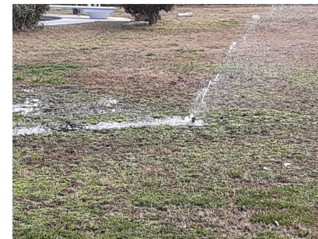
Figure 4. Waste treatment system impact-type sprinkler for distribution of treated waste. The dog has also broken the sprinkler head, causing added water problems.
