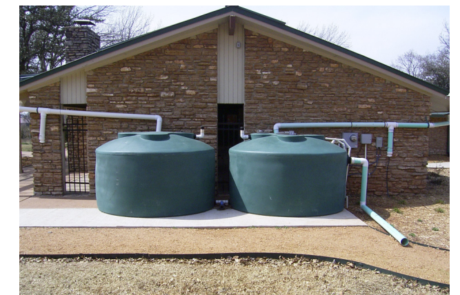
Figure 5: Rainwater harvesting system capable of capturing 2,200 gallons at the Xeriscape Gardens in Edmond, Oklahoma.
