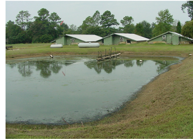
Figure 5. Alligator wastewater storage pond.
