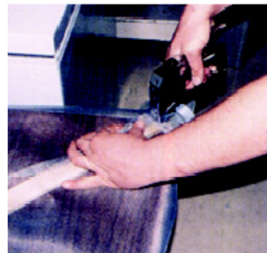
Figure 9D. Anchor trap top between screening and wood lath and staple in place.
