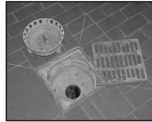
Figure 8. Floor drain and dairy brick flooring surface.
