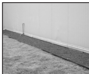
Figure 7. Pebble rock strip around production facility.
