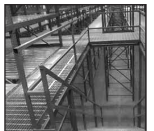
Figure 2. Overhead catwalks must not allow particles to fall through into processing areas, also, adequate kick guards should be included to prevent particles from being kicked into adjacent processing areas.
