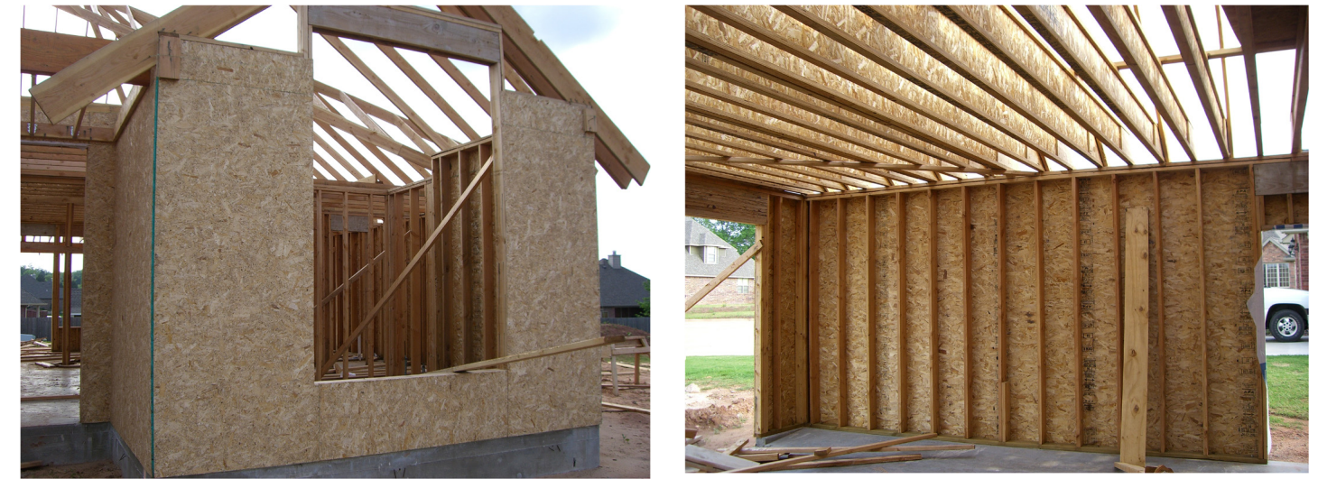
Figure 3. Applications of OSB as siding and I-joist
