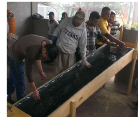
INSTALLING LATH
