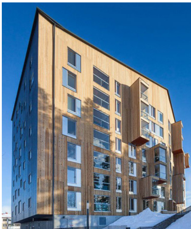
Figure 1. An example use of CLT in a seven stories tall building (source: www.bing.com ).
