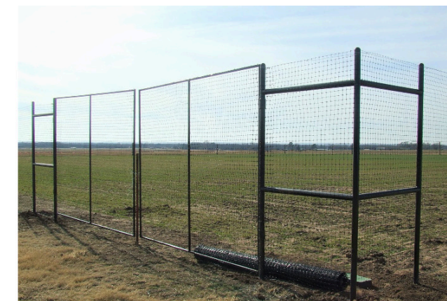
Wildlife exclusion fence. It is 8 feet tall.
