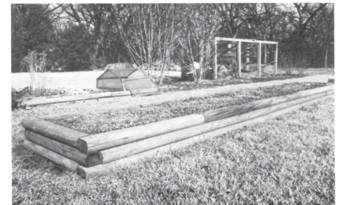
B. Reinforcing Rods Hold Timbers Together.
