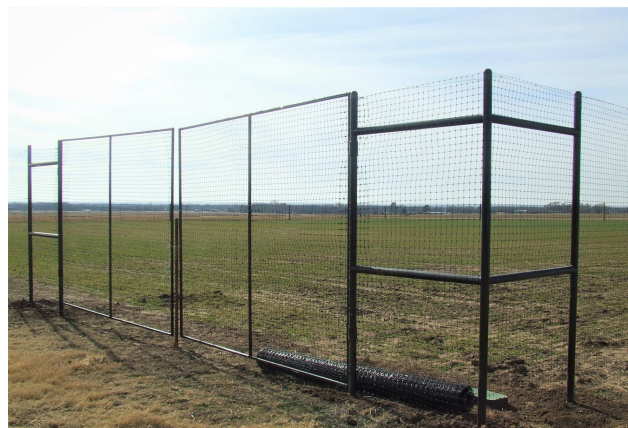
Wildlife exclusion fence. It is 8 feet tall.
