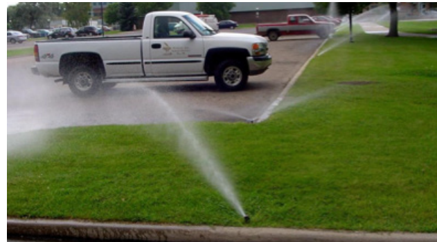
Figure 5. An irrigation zone with a mix of rotors and fixed spray sprinklers.
