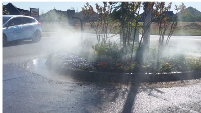
Figure 2. Sprinkler heads with excessive or high pressure causing misting of irrigation water.
