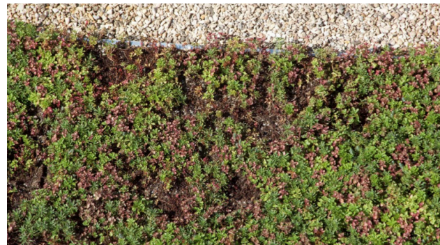
Figure 7. A dry area due to poor sprinkler distribution and uniformity.
