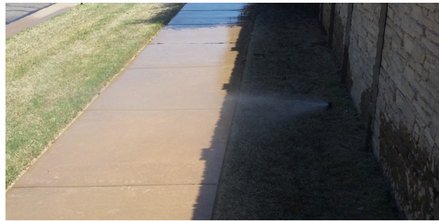
Figure 1. Sprinkler head spraying a sidewalk.
