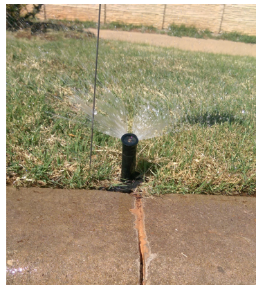
Figure 2. Sprinkler heads with excessive or high pressure causing misting of irrigation water.
