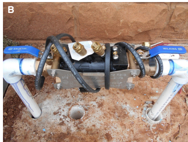
Figures 7a and 7b: Backflow preventers are designed to keep irrigation water from flowing back into the pipes used for drinking water. A pressure vacuum breaker (top) and a reduced pressure principle assembly (bottom) are two common backflow devices in Oklahoma. Note that both of the green- or blue-handled valves are aligned with the pipe. This is the fully open position. Photos courtesy of the City of Oklahoma City.
