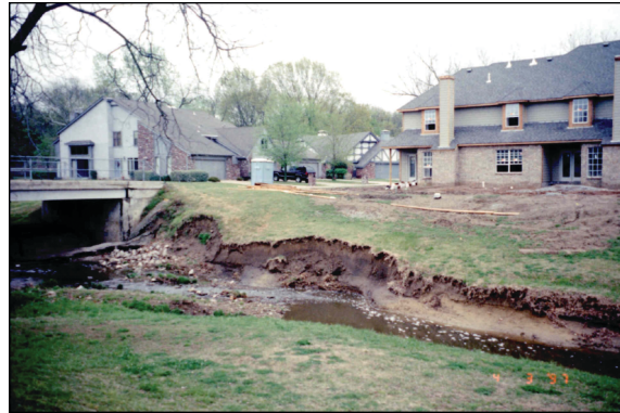
Figure 1. Construction and removal of riparian vegetation cause stream bank erosion.
