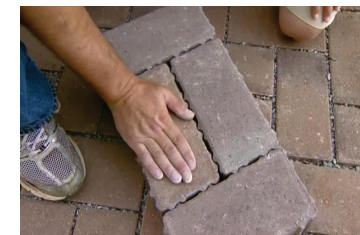
Figure 2. Pervious pavers: Consider the installation of pervious hardscapes that allow water to infiltrate rather than run off.
