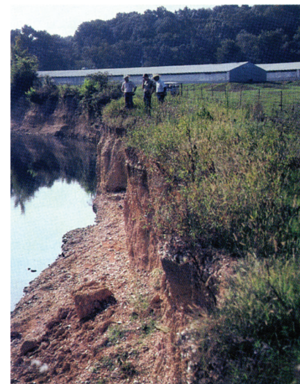
Figure 5. This high cut bank is the sign of an unhealthy, unraveling stream channel. The channel is being widened as the stream seeks to meander. Once a stream has been degraded this severely, there is little a landowner can do about it. (Photo credit: Mitch Fram)
