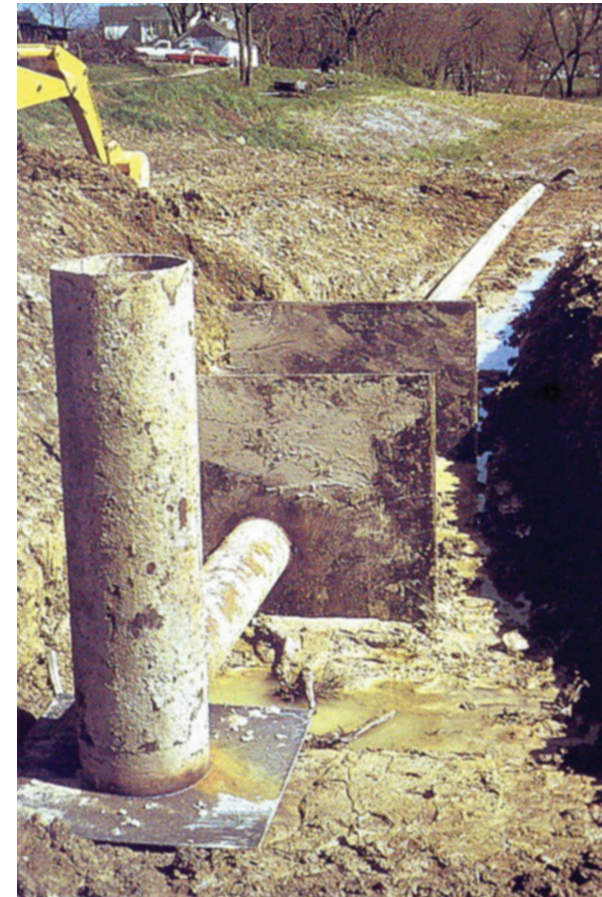
Figure 6. A smooth steel drain being installed in the early stages of dam construction. Proper drain installation involves proper slope, anti-seep collars (two shown here) and thorough compaction of each soil layer using a “jumping jack.” Beware of corrugated steel pipe: it is often short-lived due to corrosion. PVC or smooth steel pipe offers longer life. Avoid steel pipe that has been used for salt water. Image courtesy USDA - NRCS.
