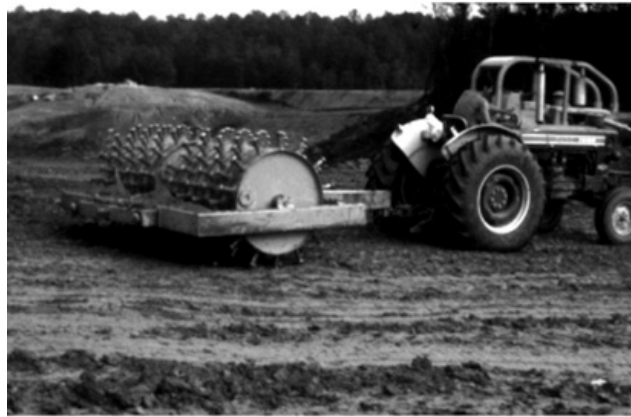
Figure 9. A sheepfoot roller can be used in compacting each lift during dam construction. Dozer tracks are a common alternative. Use of smooth rollers should be avoided. Image courtesy Alabama Cooperative Extension Service.
