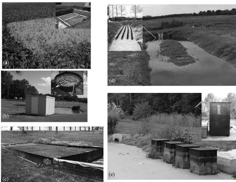
Figure 7.1 Photographs of example phosphorus removal structures: (a) blind inlet with inset showing drainage pipes prior to completion; (b) pond filter with inset showing phosphorus sorption material bed located inside building; (c) confined bed runoff structure; (d) ditch filter with inset showing drainage pipe installed prior to addition of phosphorus sorption material; (e) storm water basin filter, with inset showing the perforated metal box containing phosphorus sorption material.
