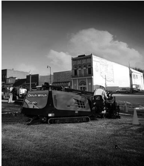
Figure 8.5. Example of a HDD drilling operation in an urban area.
